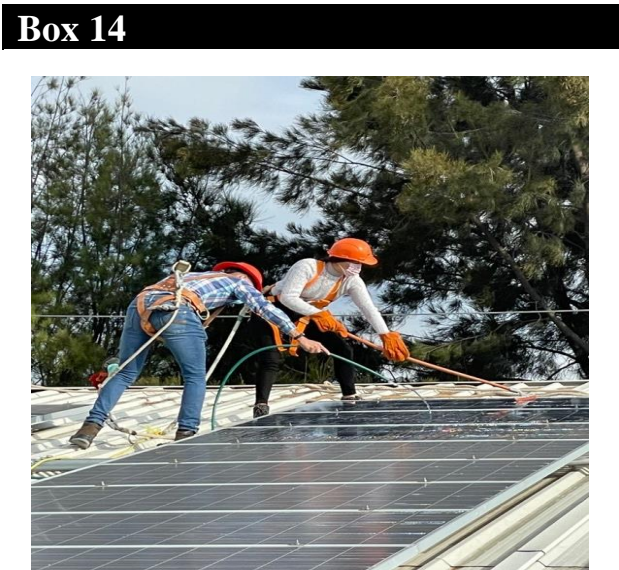
Figure 7 Maintenance activities on the roof of photovoltaic power sources system
