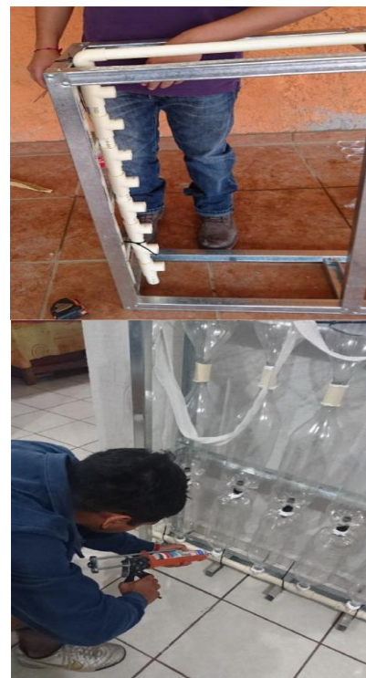
Figure 3 Placement of bottles for catchment wall [by the authors]
