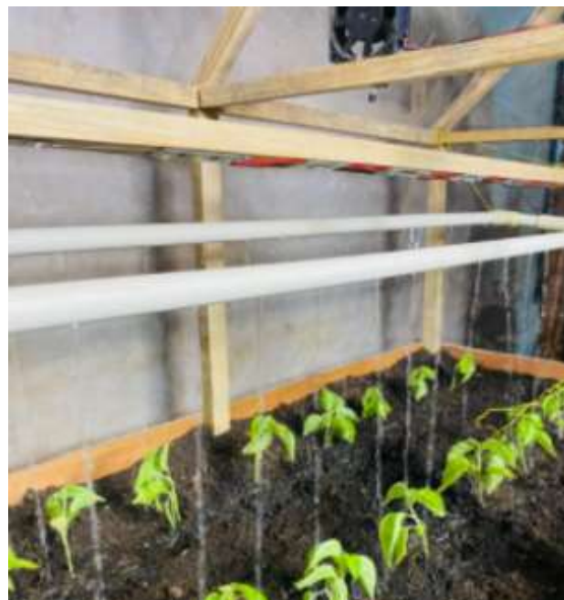
Figure 25 Irrigation system working properly
