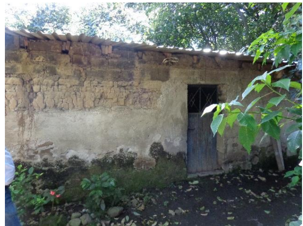
Figure 9 Adobe wall and roof with wooden beams and corrugated sheeting in Tochimilco, Puebla Source: (Vázquez, 2019)
