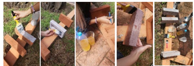
Figure 6 Application of waterproofing in brick Source: own elaboration
