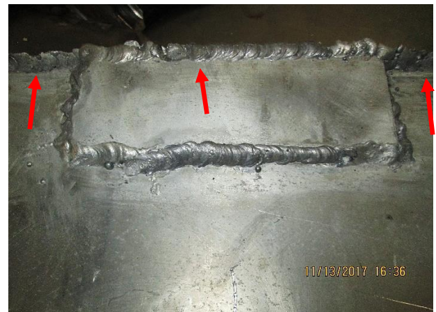
Figure 8 The image shows 7X that the fracture grew along the weld seam Source: own work [Canon powershot A3400IS]
