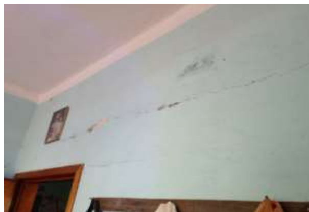
Figure 7 The longitudinal fault is seen in the image at the top Source: Faculty of Architecture BUAP, 2017
