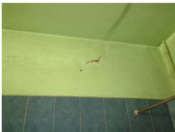
Figure 5 Bathroom of a house where the bending perpendicular to the plane of the adobe wall is shown Source: Faculty of Architecture BUAP, 2017
