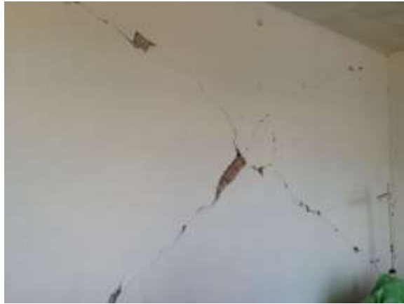
Figure 10 It fails by bending perpendicular to the plane of the wall by static instability of the segments caused by the rigidity of the upper dala Source: Faculty of Architecture BUAP, 2017
