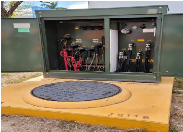
Figure 2 225 three-phase transformer (T2) (kVA)
