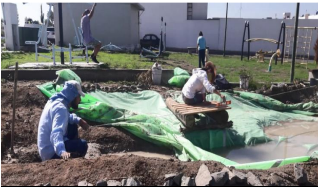
Figures 7 Construction process of the biopond at BUAP Residential Complex Source: Alonso (2019)
