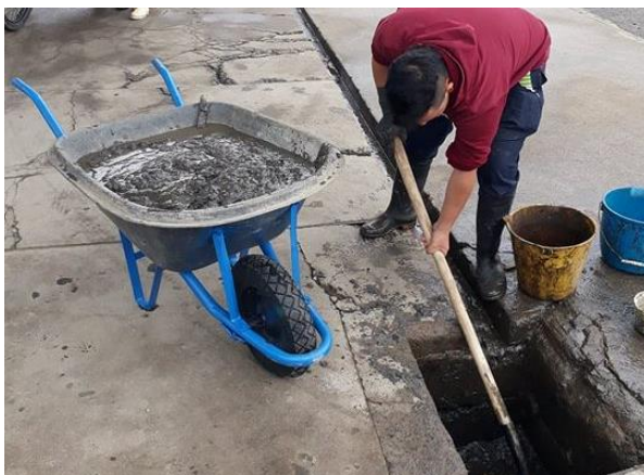
Figure 2 Extraction of sediments from the grease trap
