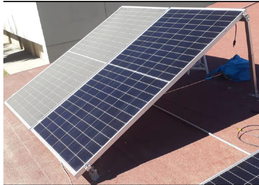
Fig.1 JaSolar modules of 410 W, dirty vs clean [Own source]
