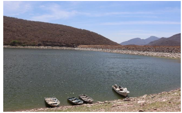
Figure 1 Basilio Vadillo Dam, Jalisco Mexico spring 2022
